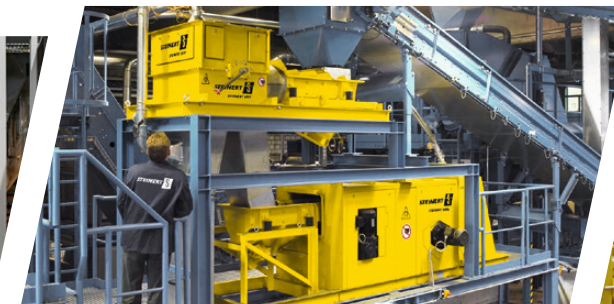
Removal of ferrous parts using STEINERT MOR
