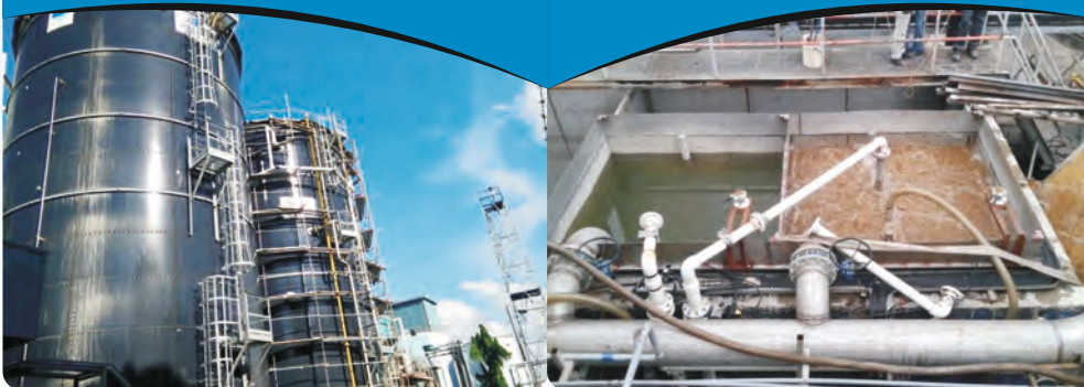
1000 M3/Day MBR Based Palm Oil Effluent Treatment Plant
