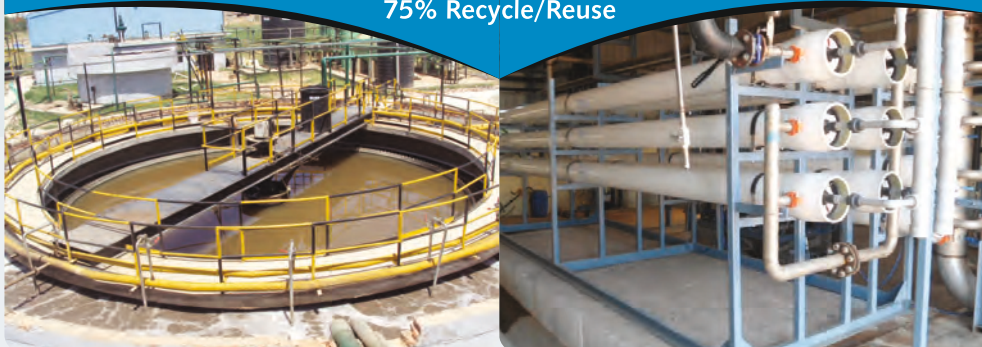
1800 M3/Day (330 GPM) Brewery Effluent Recycling/Reuse Plant 75% Recycle/Reuse
