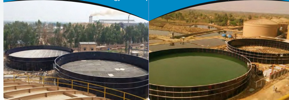
1500 M3/day Waste Water Treatment Plant based on Anaerobic Hybrid Reactor (AHR) Technology and Sequential Batch Reactor (SBR)
