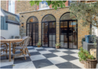
YES GLAZING SOLUTIONS (FULHAM PROJECT)
