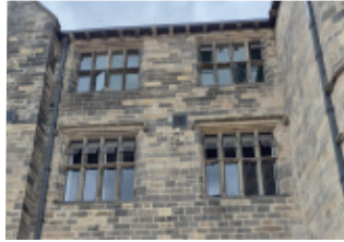
TOUCHSTONE GLAZING SOLUTIONS (ROCHDALE TOWN HALL)
