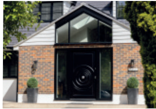
YES GLAZING SOLUTIONS (WESTERHAM PROJECT)
