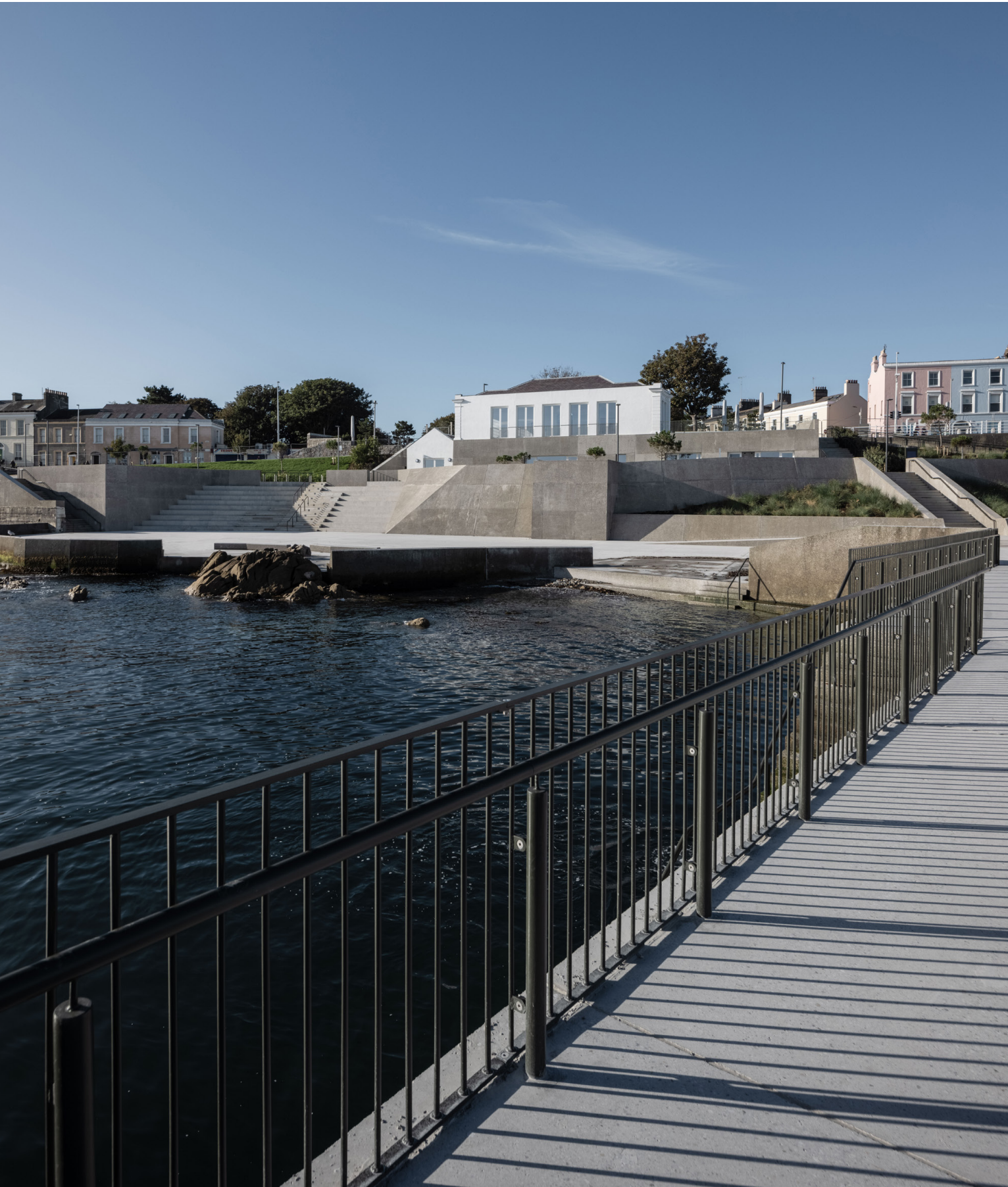
VIEW FROM JETTY TOWARDS FOLDING CONCRETE WALLS, STEPPED AMPHITHEATRE AND PAVILION WITH PEOPLE'S PARK IN BACKGROUND
