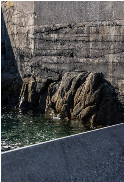
PALIMPSEST OF SEA ROCK, CONCRETE SEA WALLS AND OVERMOUNTED CONCRETE
