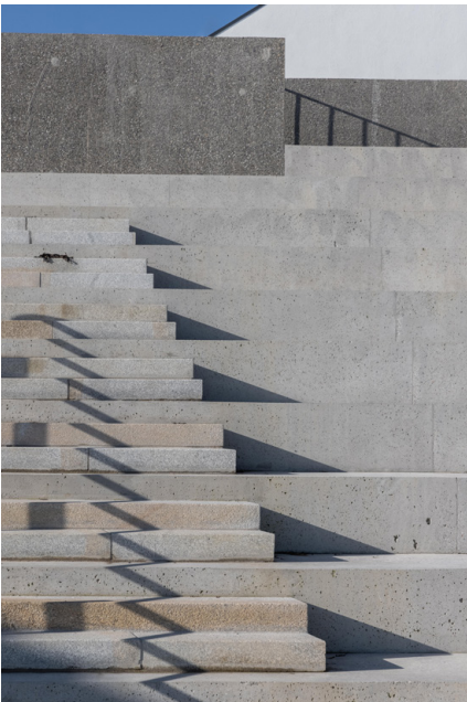
DETAIL OF GRANITE AND CONCRETE AMPHITHEATRE STEPS
