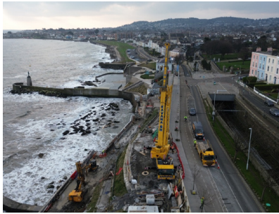
ADDITIONAL ACCESSIBILITY WORKS FOR COMPLETION SUMMER 2024 - DRONE AERIAL VIEW
