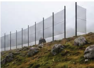
PLASTIC MESH INSTALLATIONS
