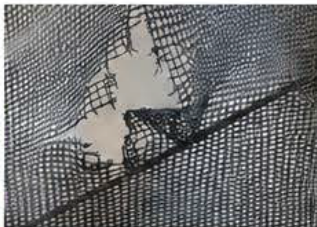
TEARING UNDER HIGH WIND
