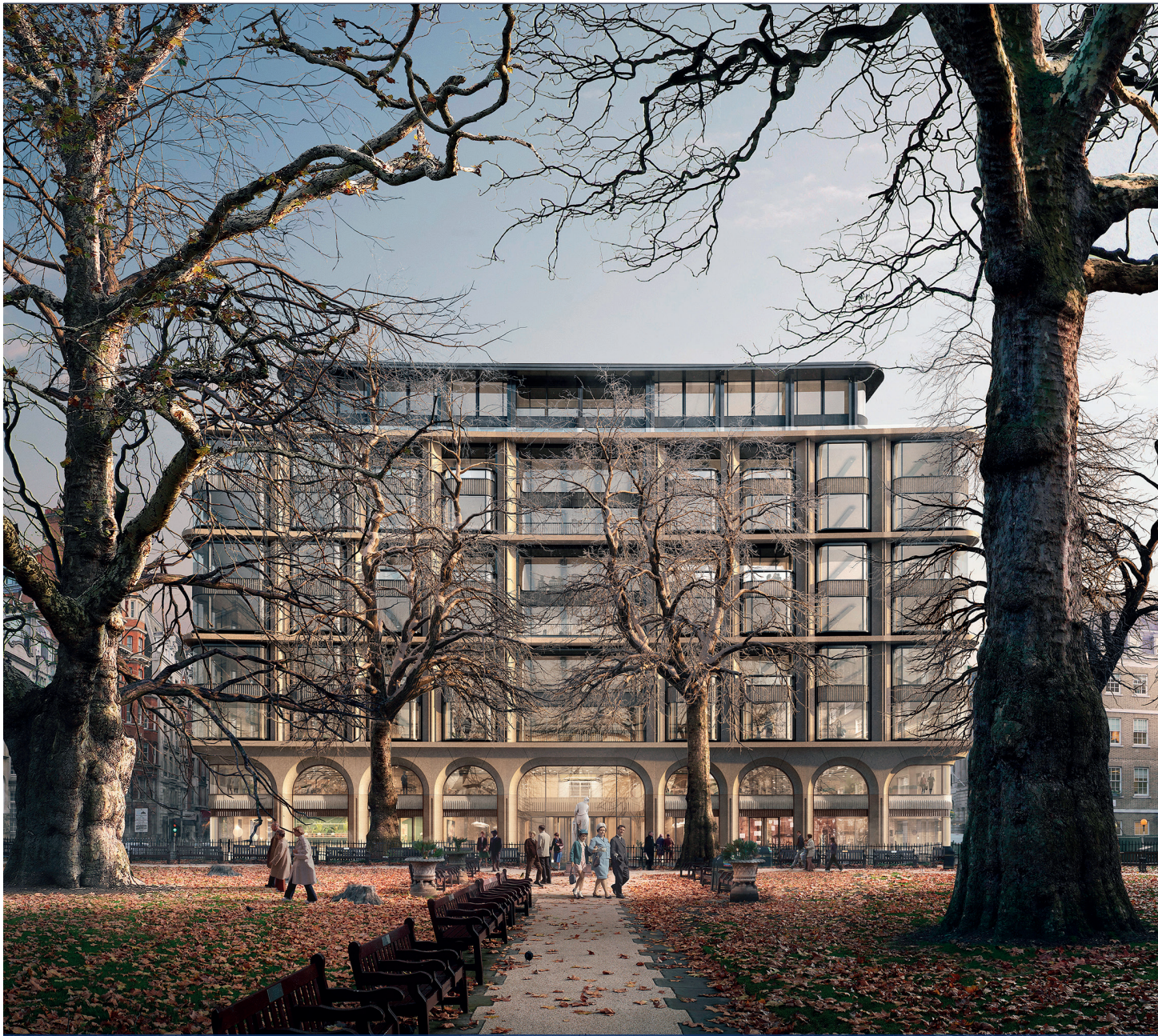
Taking shape: CO-RE is working on the Lansdowne House office development in Mayfair, due to be completed in 2027
