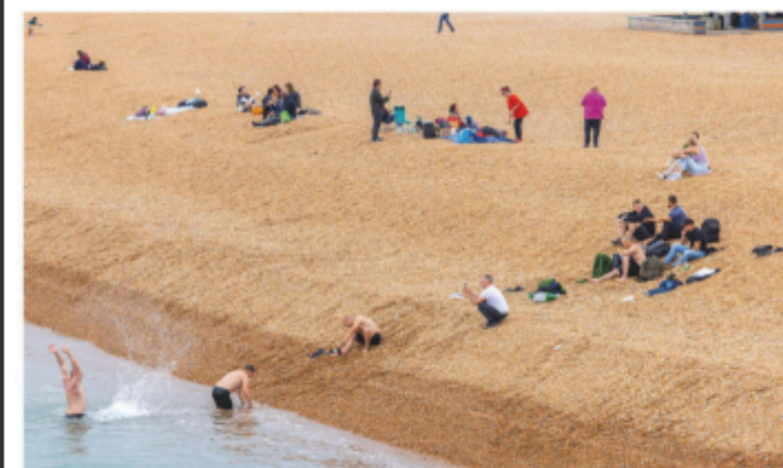
The shingle on the beach has been moved and refilled to offer protection from storms.
