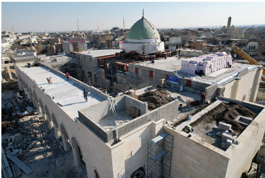
Four religious monuments, 124 houses and 404 classrooms were rebuilt as part of the programme
