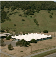
Herzog & de Meuron and EHDD to create Eames design museum in 1960s warehouse
