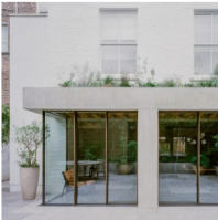
DF_DC adds concrete-framed extension to London home
