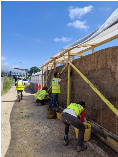
Global Generation is using waste earth to create a cob classroom. Photo by Global Generation
