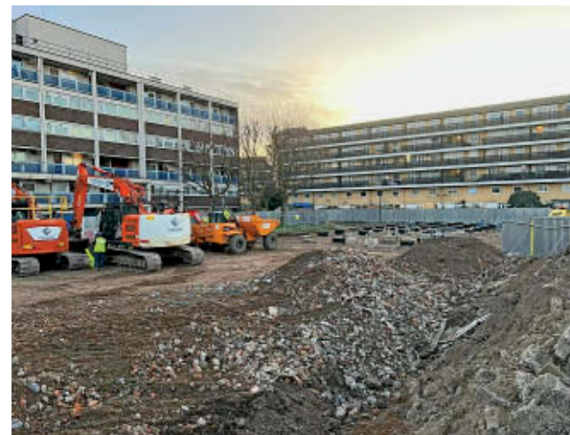
From top: John Dickson, 62, bought his flat in south London through the policy but now faces a bill of up to £35,000 to pay for improvement works; the building of new council homes on the Bells Gardens Estate in southeast London has stalled for lack of money
