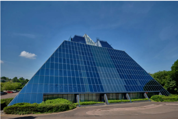
The Stockport Pyramid at Junction One of the M60 designed by Christopher Denny from Michael Hyde and Associates (completed 1992) Source: Shutterstock/iron bell
