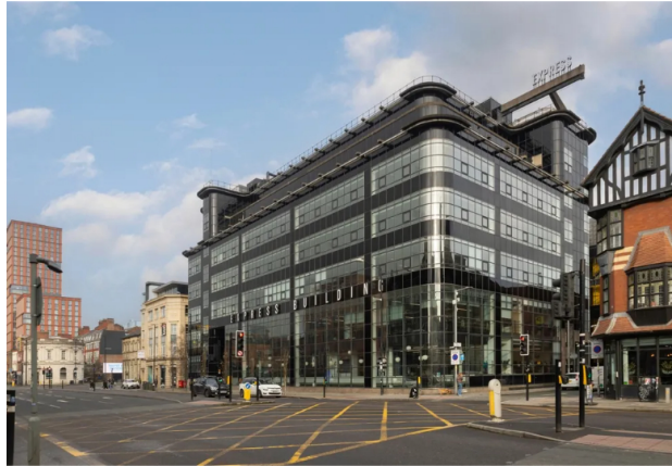
The Daily Express Building in Manchester which was given an overval by MHA Architects in the mid 90s
