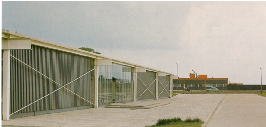
The Reliance Control factory was Team 4's biggest project. Photo by Norman Foster
