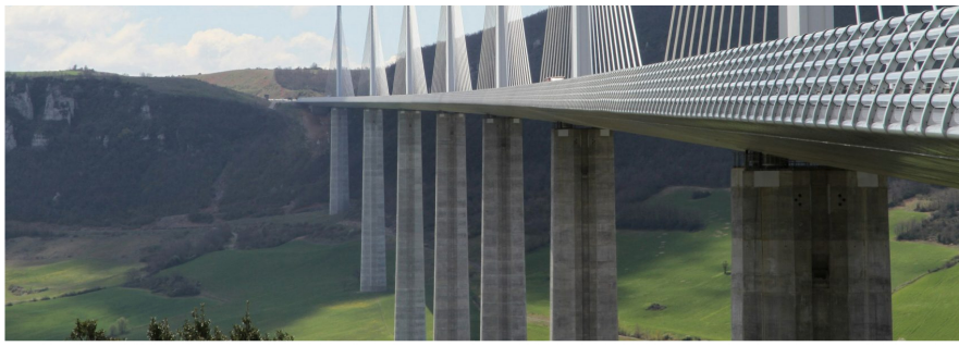
Completed in 2004, the Millau Viaduct in southern France remains the tallest bridge in the world. Photo by Luca Onniboni
